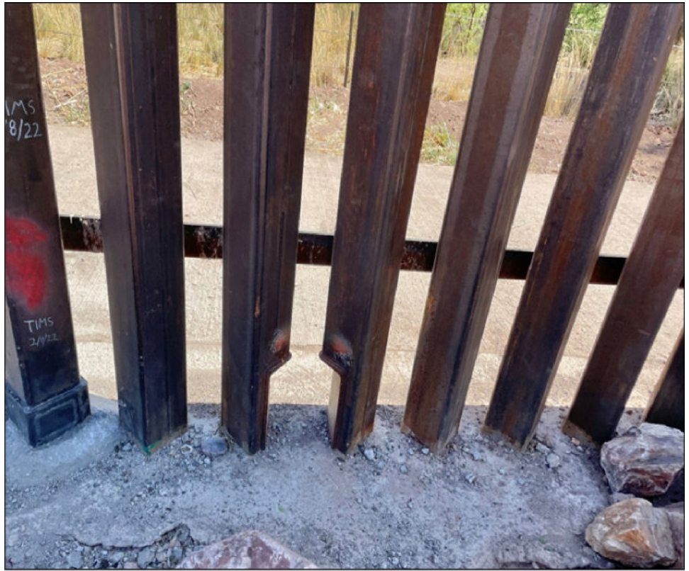
Figure 8: Border Barrier with a Small Opening (8½ by 11 inches) for Animals (May 2022)
