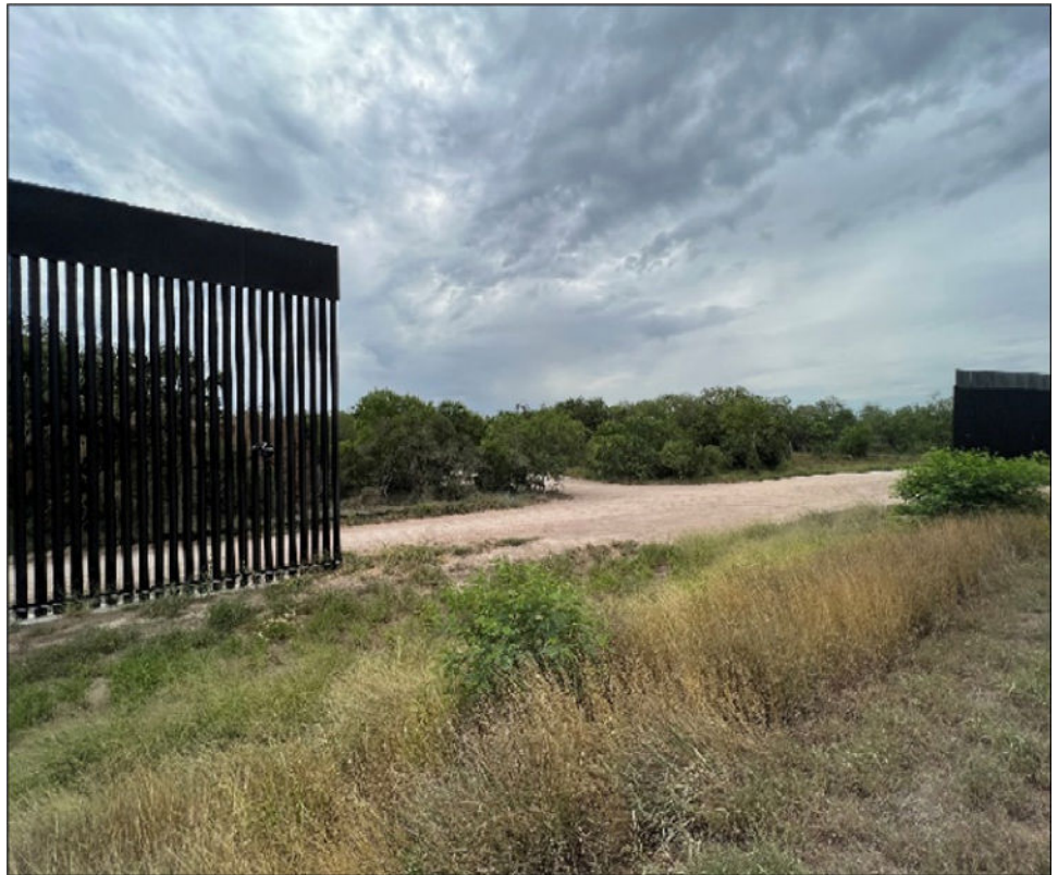
Figure 12: Opening Between Installed Panels in Texas (July 2022)
