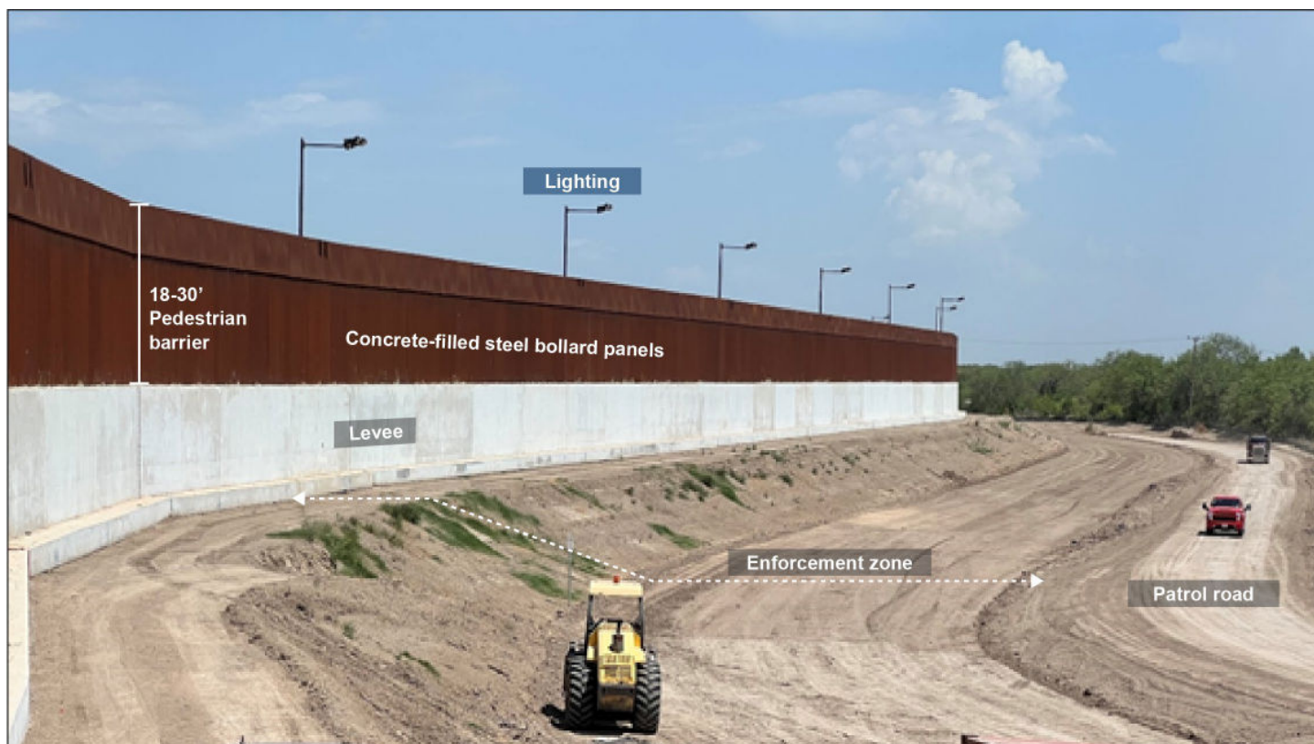
Figure 4: Border Wall System Program Components, Including Barrier atop a Levee, Rio Grande Valley, Texas (July 2022)
